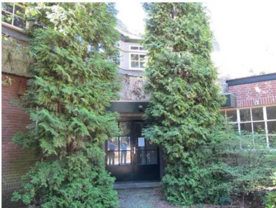
Entree in de noordgevel. (MAB, 2011)
